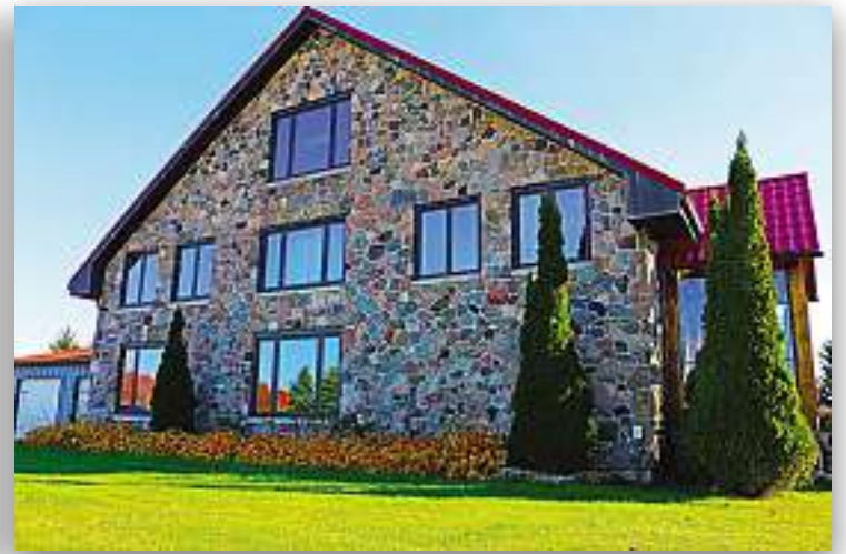
Former owner John Herman completed the exterior of this timber frame house in 1996 using stone collected from old barn foundations
