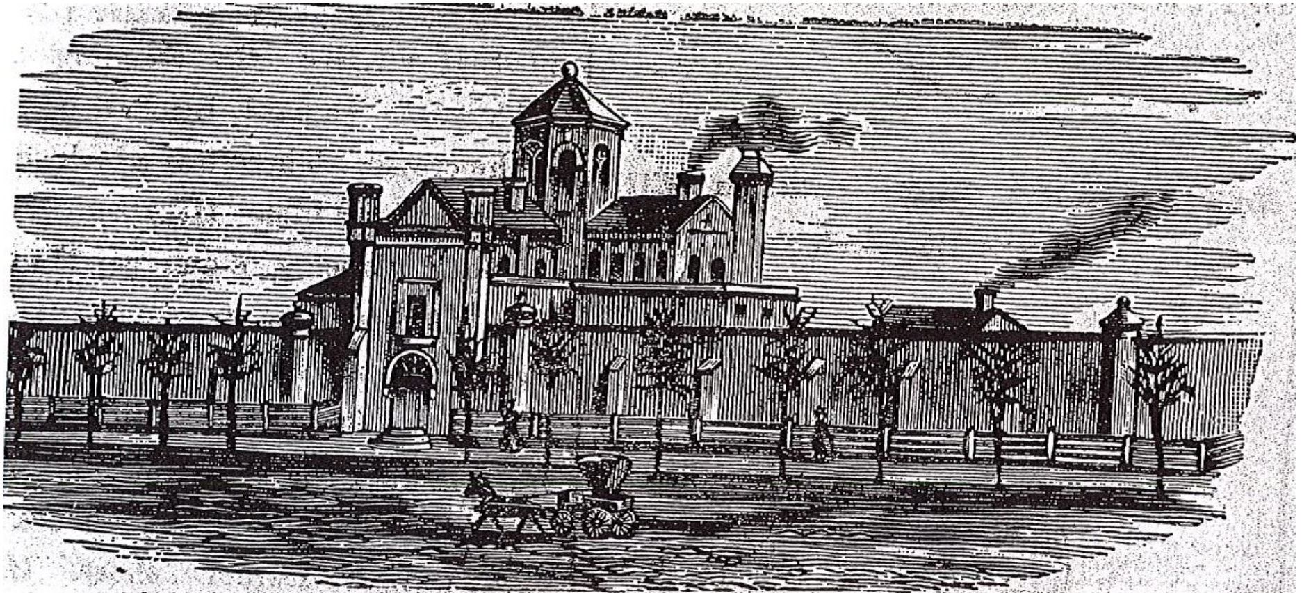
THE GAOL LOOKING NORTH, (The Cook Execution took place just East of the Main Entrance )
